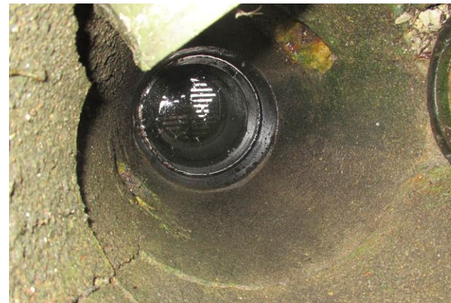
Betonbrønd i mindre god stand.
